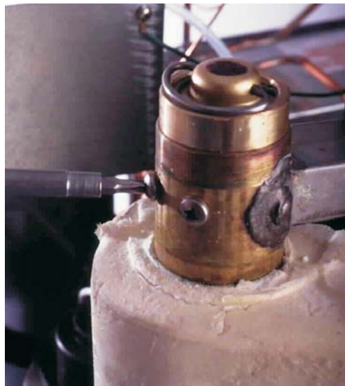
Remove Two Screws
